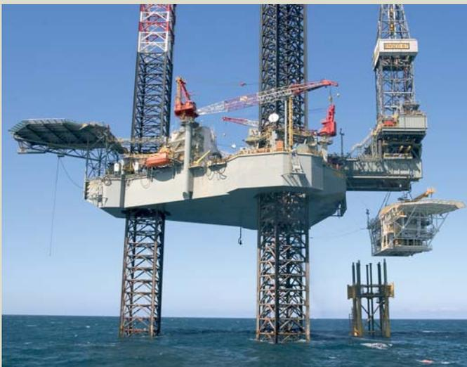
The **Ensco 67** jack-up drilling rig lifting the 498 tonne deck component of the Cliff Head "A" Platform onto the platform jacket.
