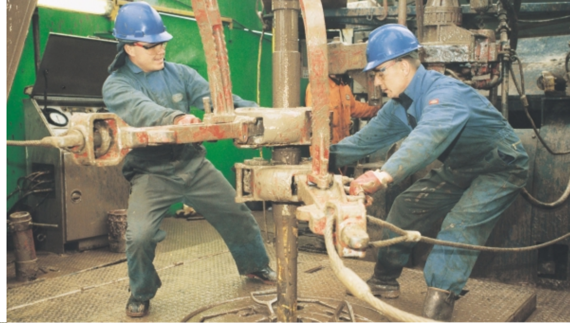
Drilling Saltfleetby-6, onshore UK.
