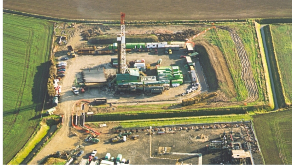
Saltfleetby-6 drill site and adjacent production facilities, onshore UK.
