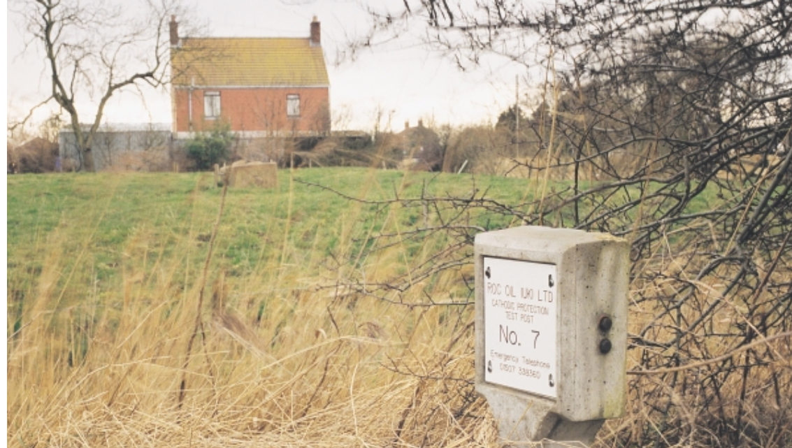
Pipeline marker post for pipeline connecting Saltfleetby to the Theddlethorpe Gas Terminal, onshore UK.
