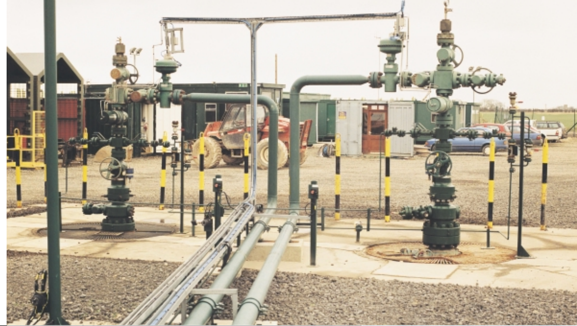
Saltfleetby Gas Field surface facilities.
