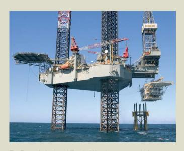
The **Ensco 67** jack-up drilling rig lifting the 498 tonne deck component of the Cliff Head "A" Platform onto the platform jacket.
